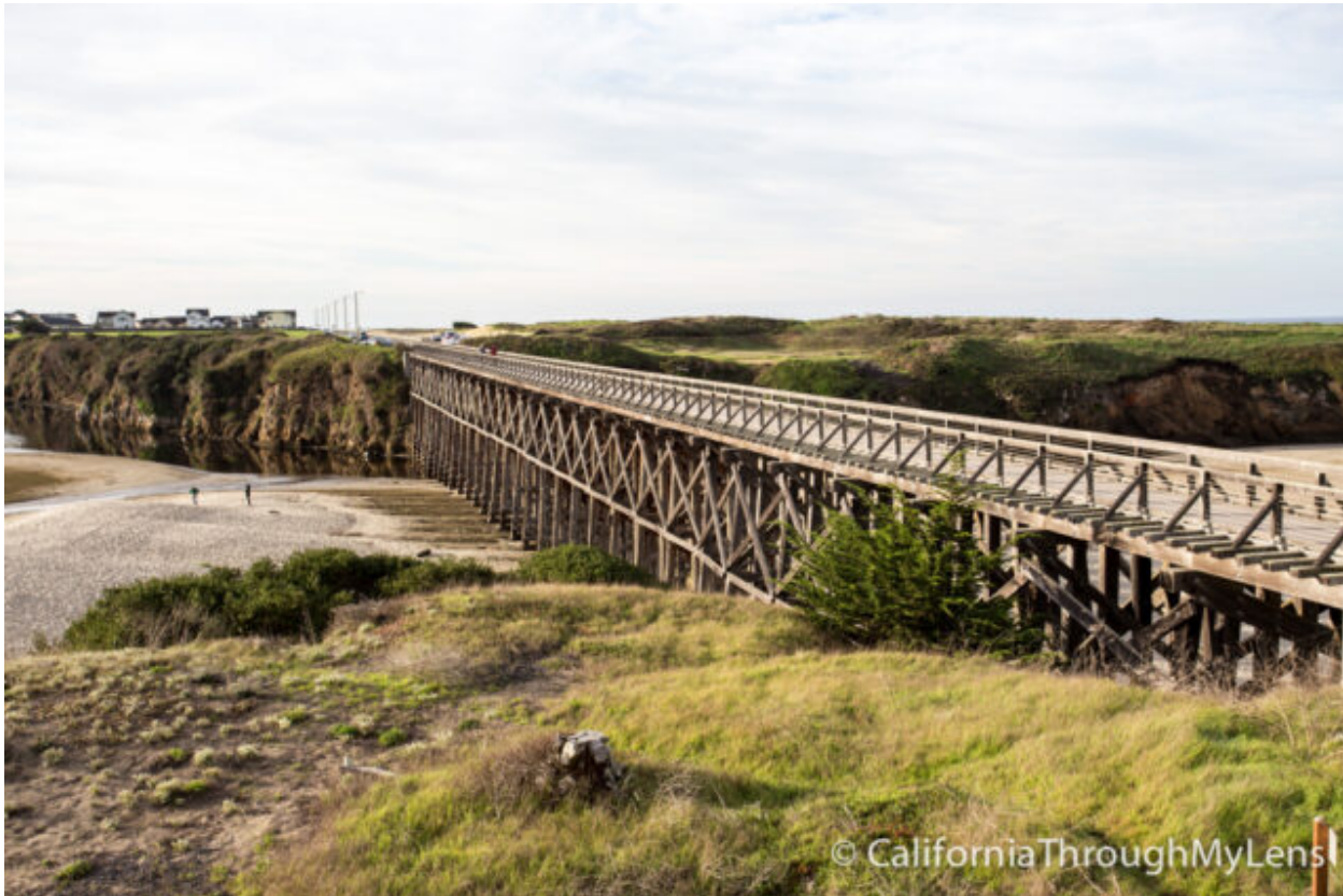
Pudding Creek Trestle — rehabilitated pedestrian/equestrian path, 2007
