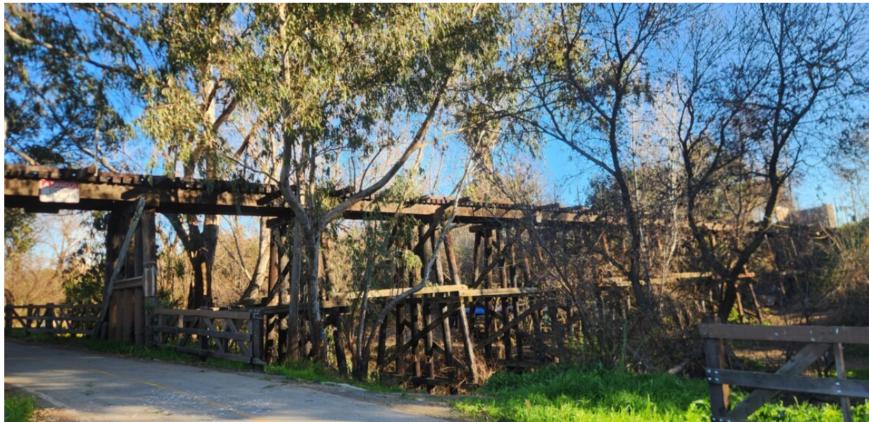
Coyote Creek Trestle — 1922 Western Pacific timber pile bent trestle
