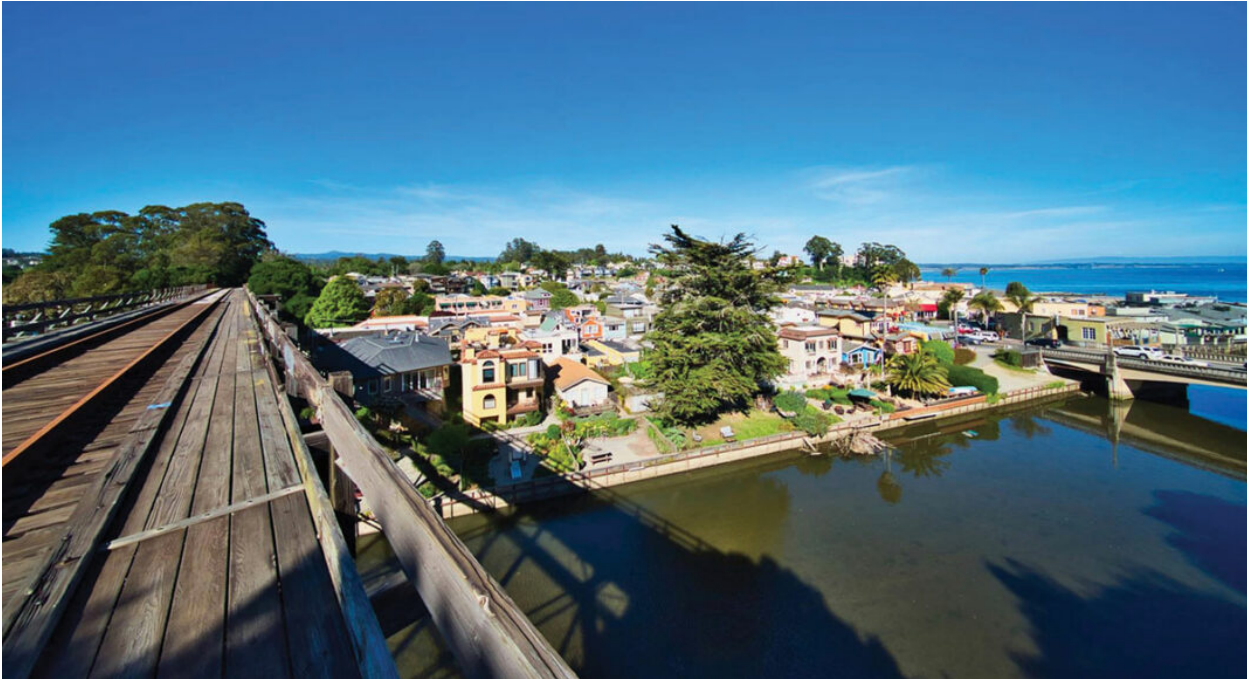
Capitola Trestle complex — crossing Soquel Creek and downtown streets
